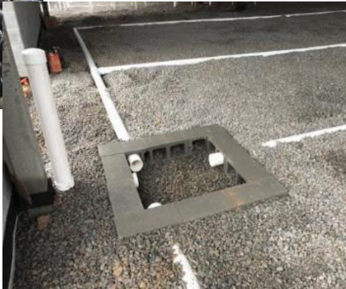
Passive Sub-Slab Venting (SSV) Systems
