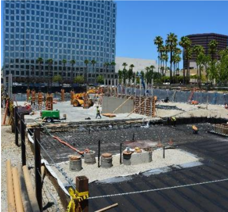
Source: EPRO Services, Inc, 2020. Used with permission.
