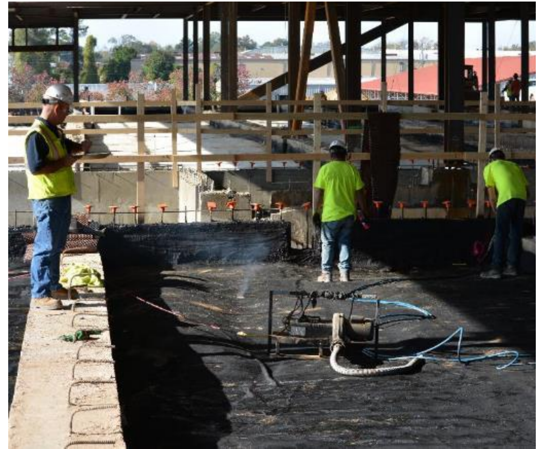
Source: EPRO Services, Inc, 2020. Used with permission.
